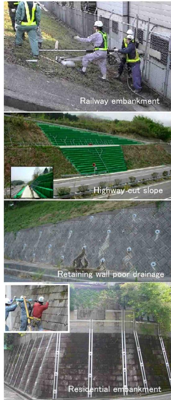
Fig.11 The applications of the pipe drain method
